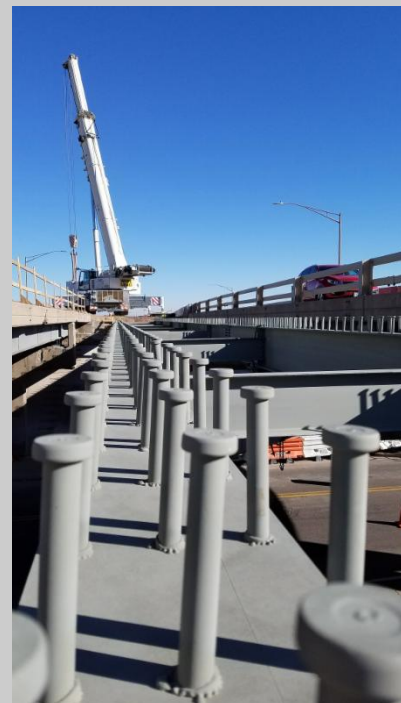
Girder work on Indiana Bridge.
