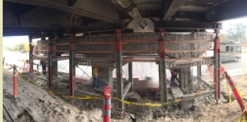
Work on the substructure of the Mesa Avenue bridge.
